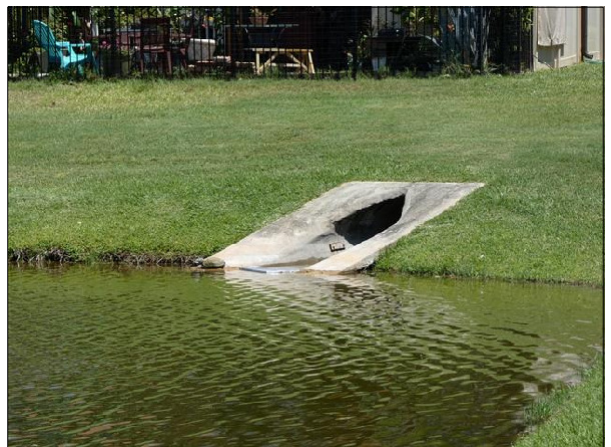
Stormwater Drainage Mitered End Section
