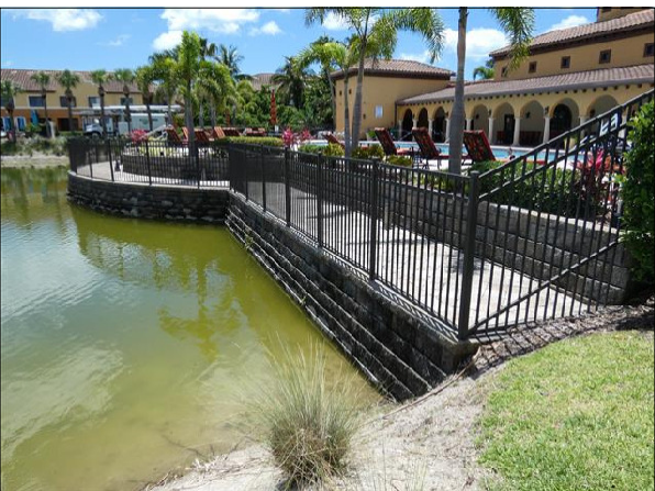
Retaining Wall at Clubhouse
