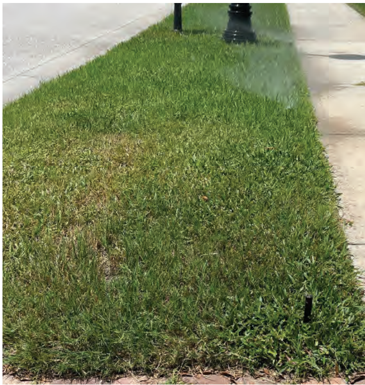
Tilted, too low, clogged nozzles
